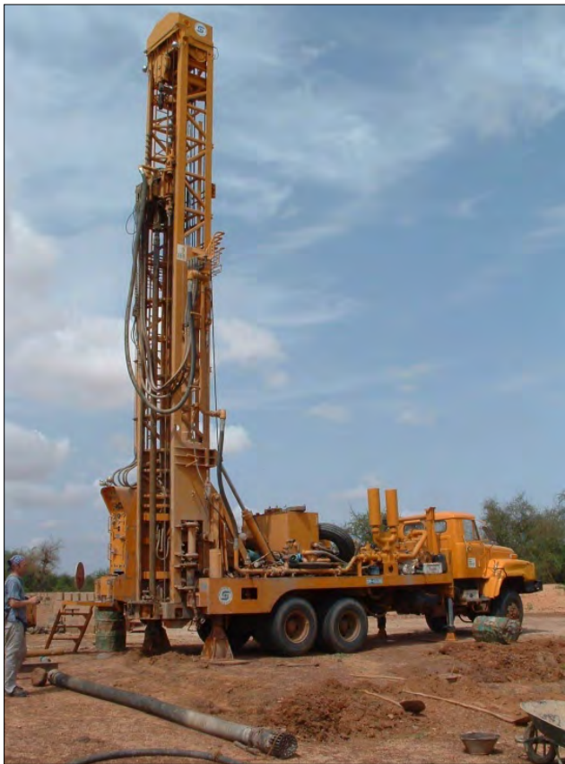
FIGURE 9. Drilling rig at one of the array elements at PS29.
