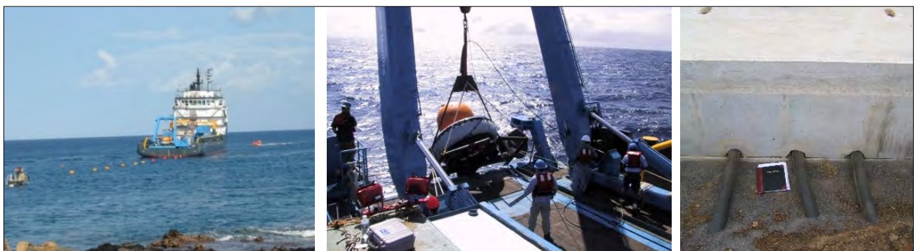
FIGURE 21. HA10 cable landing (left). Node deployment (centre) and detail of cable conduits exiting the onshore splice pit (right).
